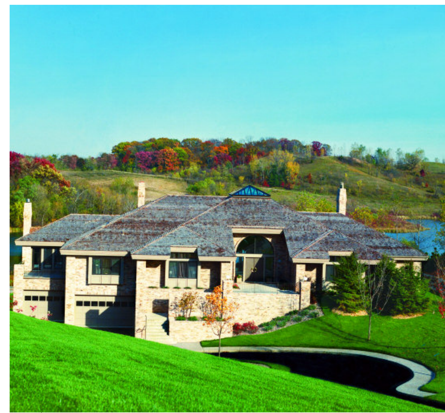
MULTIPLE LEVELS EXPLOIT THE UNIQUE ELEVATIONS OF THIS 8,000-SQUARE-FOOT BRYANT LAKE, MINNESOTA HOME, CROWNED WITH A SKYLIGHT TO ACCENTUATE THE FOYER.
